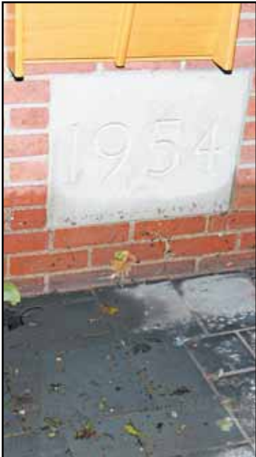
Moonachie Mayor Dennis Vaccaro's first assessment of Borough Hall. The force of the water blew out one of the door windows. Water level still visible on the 1954 cornerstone. Borough engineer indicates that the force of the water twisted the back door.
