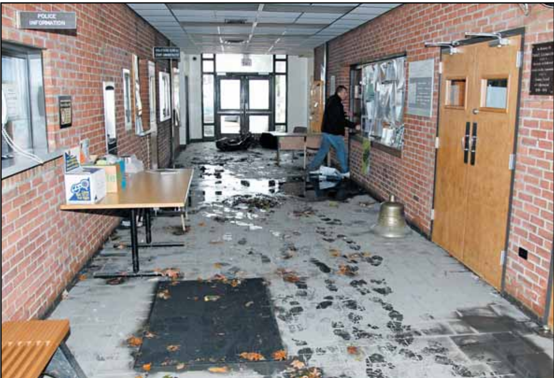
Moonachie Mayor Dennis Vaccaro's first assessment of Borough Hall. The force of the water blew out one of the door windows. Water level still visible on the 1954 cornerstone. Borough engineer indicates that the force of the water twisted the back door.
