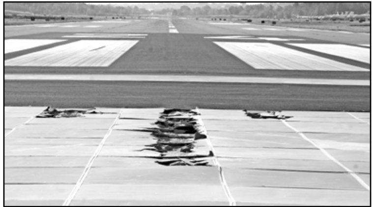
Damage done to the EMAS during the October 25, 2006 incident affected about 15 panels.
