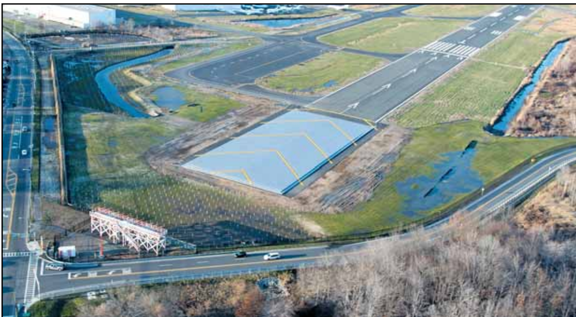
PA Installs 2nd Arrestor Bed at TEB, February 2012
