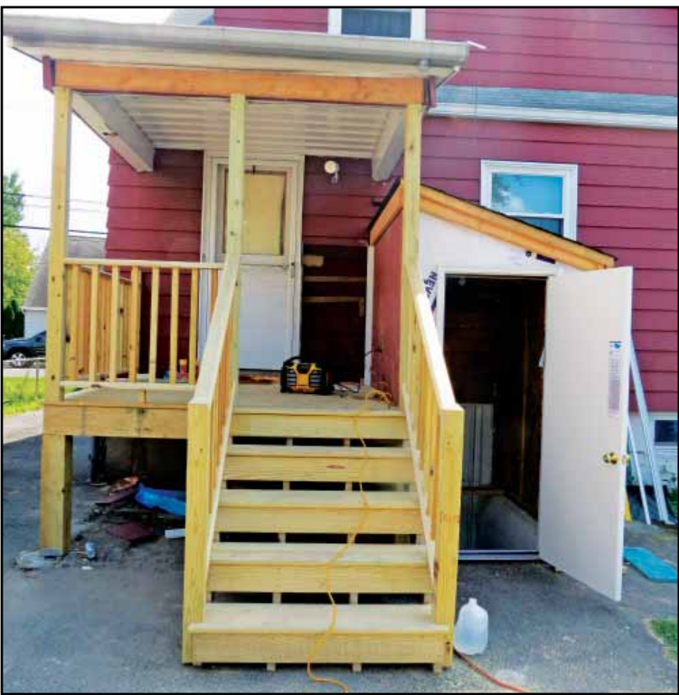
On August 5, 2015, Rebuilding Together Bergen County deconstructed a porch which was rotting from water damage in Little Ferry, NJ. The family of six sought help through the Long Term Recovery Center after Sandy. The porch was rebuilt and included the enclosure over the exterior basement steps. The spindle/post railing replaced the solid wall construction that kept water and snow in, and probably contributed to the wood rot/buckling. Bottom photo of newly constructed porch on August 21. For more information, go to: www.rebuildingtogetherbergen.org/ Photos by Thom Mongell. ###
